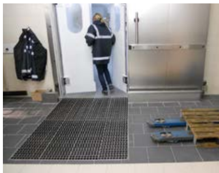
Entrance areas to deep-freeze stores
